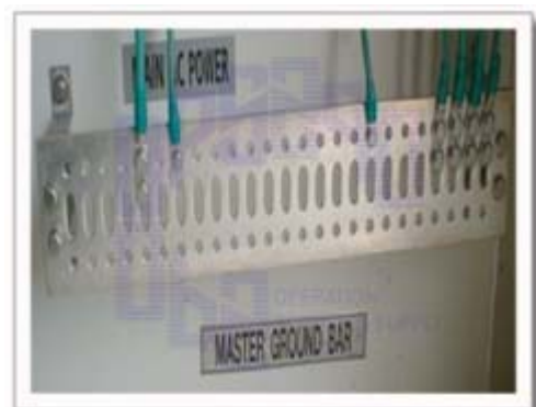
BUS BAR/GROUND BAR
